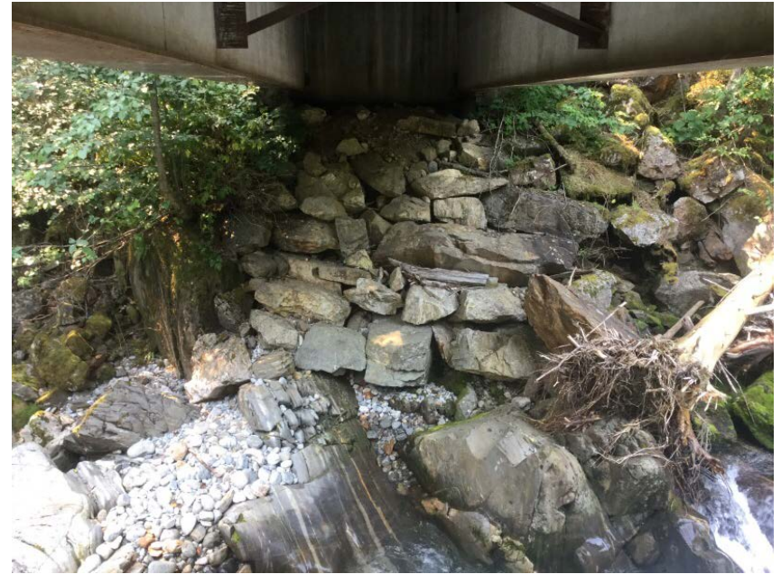
Right Bank Abutment when facing downstream
