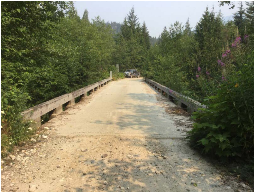
Approach from Right Bank when facing downstream
