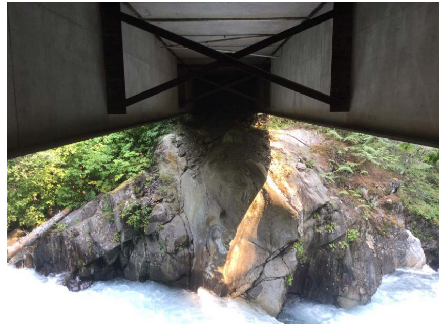
Approach from Left Bank when facing downstream
